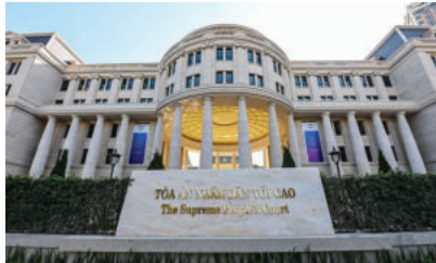
Third party liability loss - new Supreme Court building construction project
