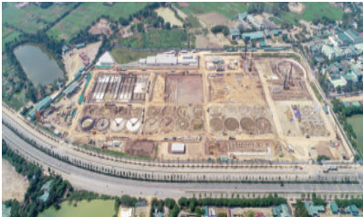
Wastewater treatment plan - flood damage
