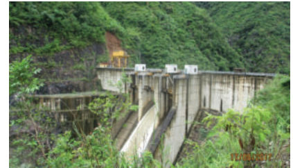
Hydropower plant - storm damage to hydro-mechanical equipment, plant electrical equipment and trash rack
